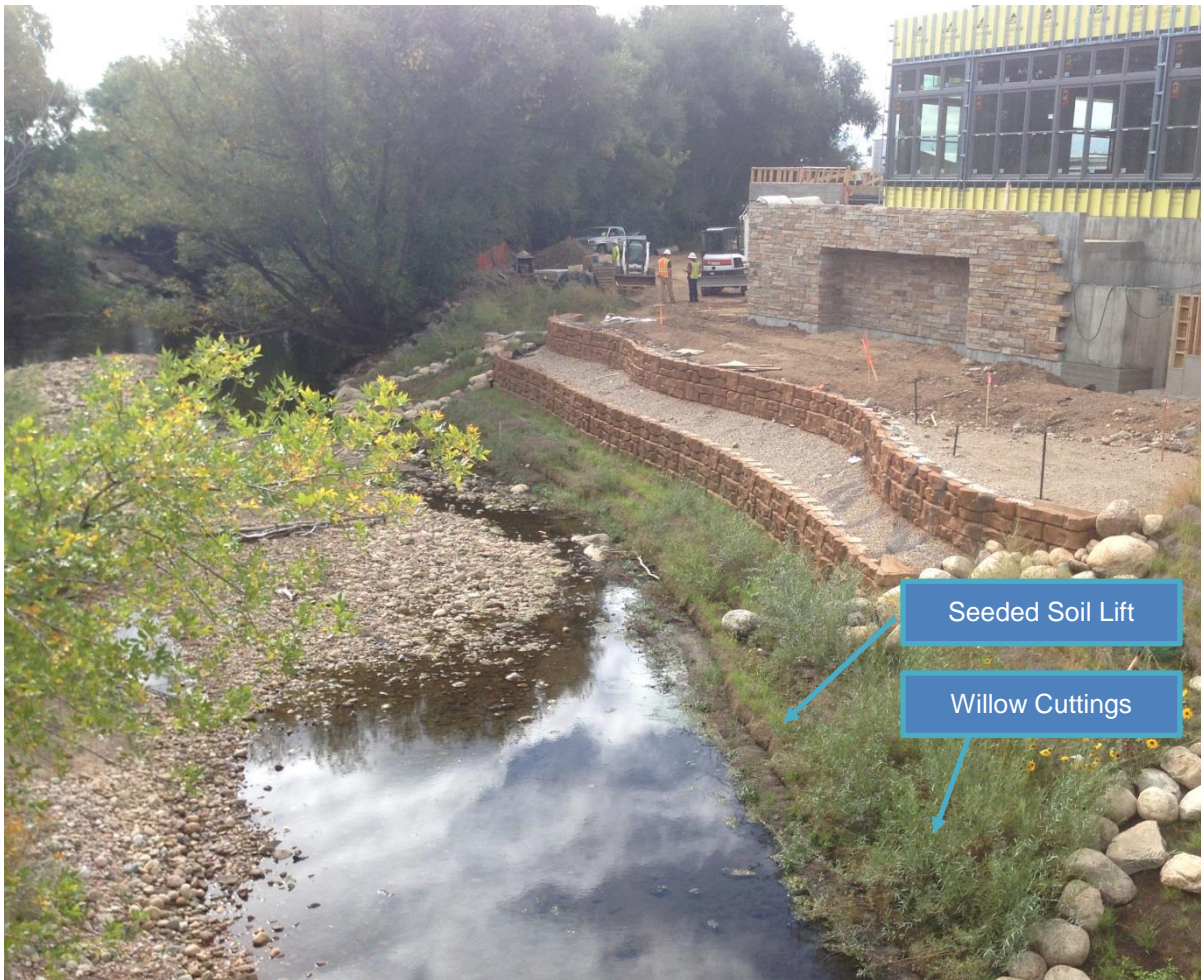
Figure 31. Vegetated soil lifts used to protect high value infrastructure on the Cache la Poudre River, Fort Collins, CO. Two seasons post-construction. From Giordanengo, J. H. Reprinted with permission.
