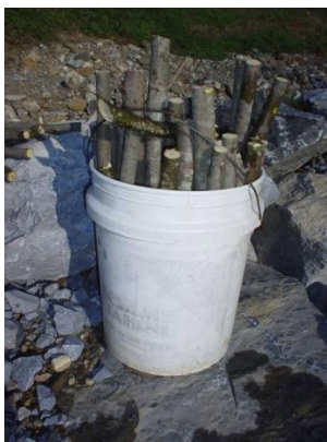
Figure 10. Willow stakes ready for installation. From Blazewicz, M. J. Reprinted with permission.
