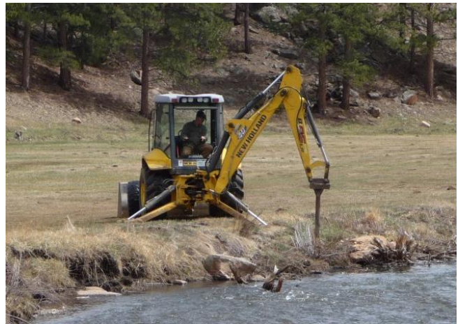
Figure 11. Mechanical stinger probing into the groundwater for willow installation on Tarryall Creek, CO. From Giordanengo, J. H. Reprinted with permission.
